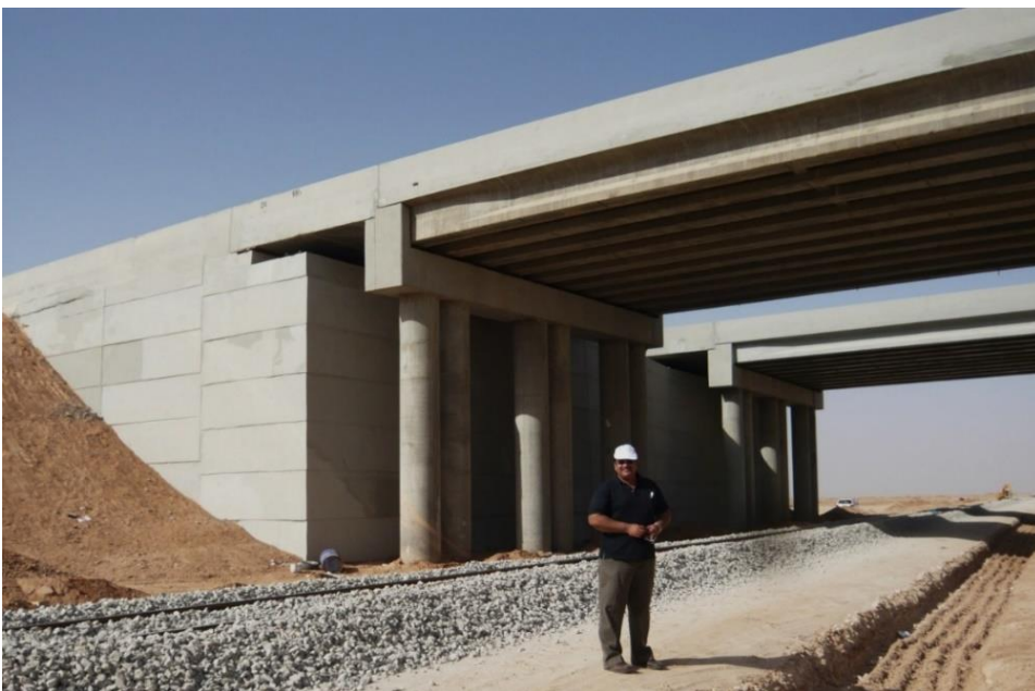
Bridge sits on separate pillars
