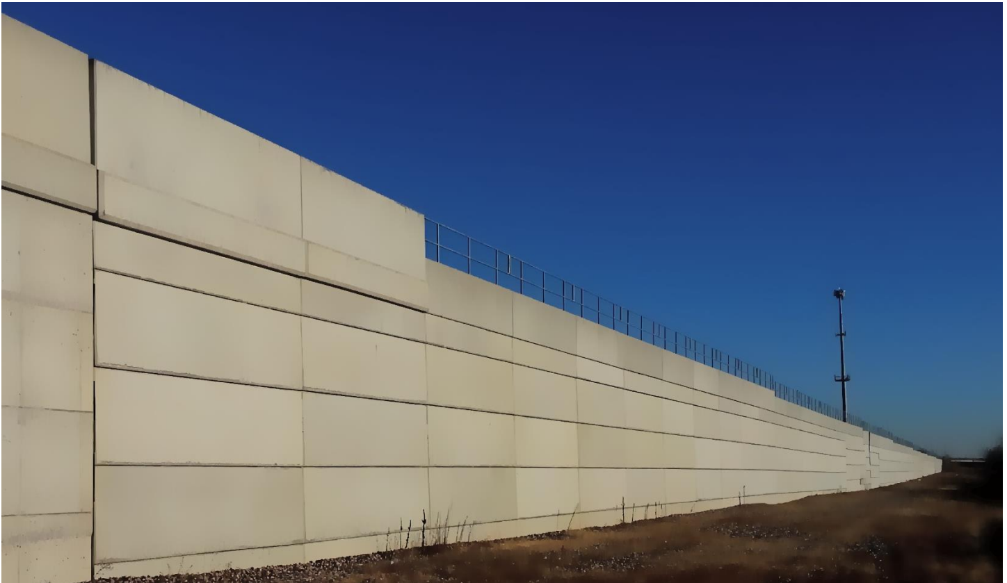
Gravity frame MAXI WALL built for BNSF in Olathe, Kansas, the flagship of MAXI PILLAR wall
